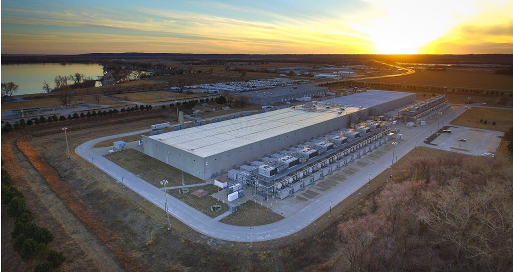
Picture two. A Google data centre in Council Bluffs, Iowa, photographed in 2017, which in this industry counts as ancient history. The ones going up now are larger.
